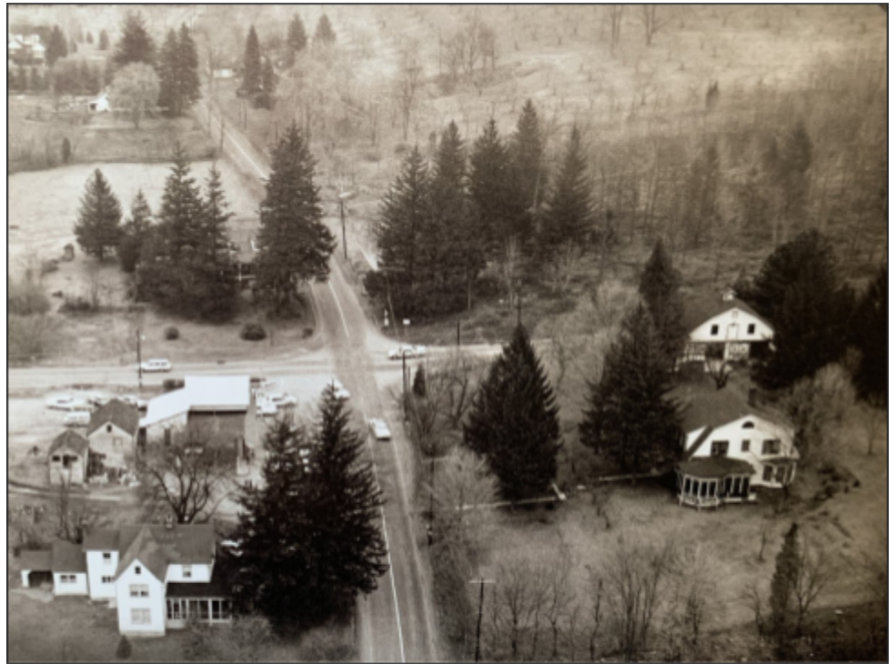
USR at the corner of Lake Street and East Saddle River Road in 1964. Photo courtesy of the USR Historical Society.
